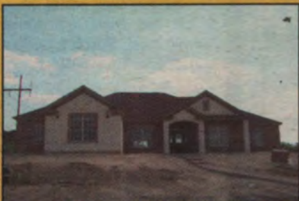
$259,900: Open kitchen, breakfast and living room. Separate formal living and formal dining are great for entertaining. 3 BR/2 BA, separate utility room, large covered back porch, beautiful entry into the front foyer.
