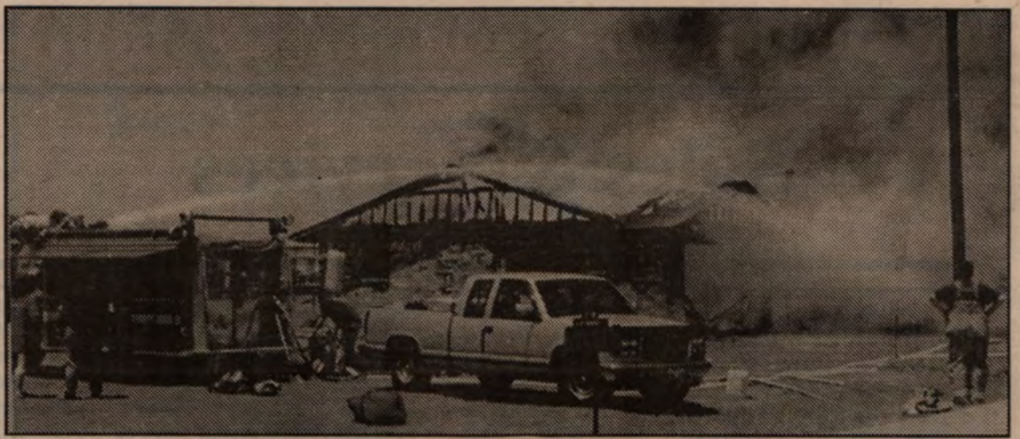
Two birds with one stone: Salado volunteer firefighters got some extra training on structure fires courtesy of Salado ISD last week. The building on Salado School Rd. which was set ablaze May 29 was recently purchased by the district and set for demolition to make room for the new middle school. Firefighters set and extinguished fires in the building throughout the day, giving them extra training for fighting structure fires. (photo by Marilyn Fleischer)
