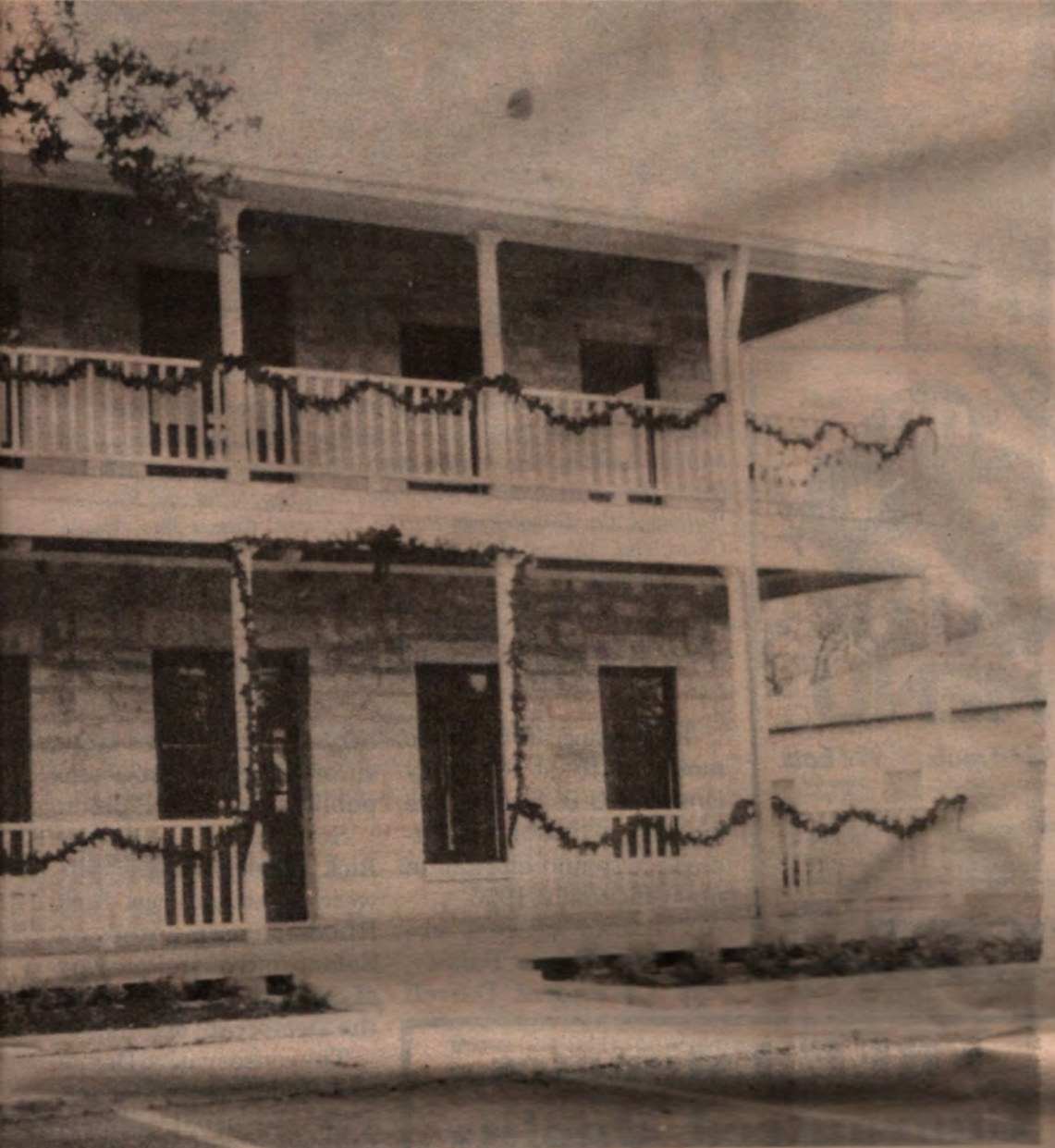
The completion of The Veranda on Salado's Main St. marks the rebirth of a fine, old Central Texas building.
