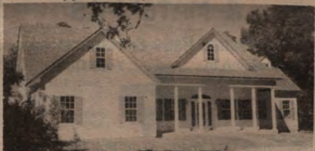
Whispering Oaks: All new home ready for landscaping to your specifications! Great floorplan with 3 BR/2 full & 2 half baths, 2 living and 2 dining All First Floor. Upstairs has guest or 4th bedroom & Bath. Beautiful interior design and finish. Pool! $279,500.
