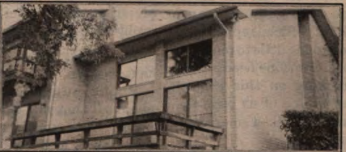
SPECTACULAR VIEW of 18th fairway from 2 of the 3 bdrm and living room of our NEW LISTING at #2 Chisholm Ridge Townhomes. Spacious kitchen with island and cabinets GALORE!
