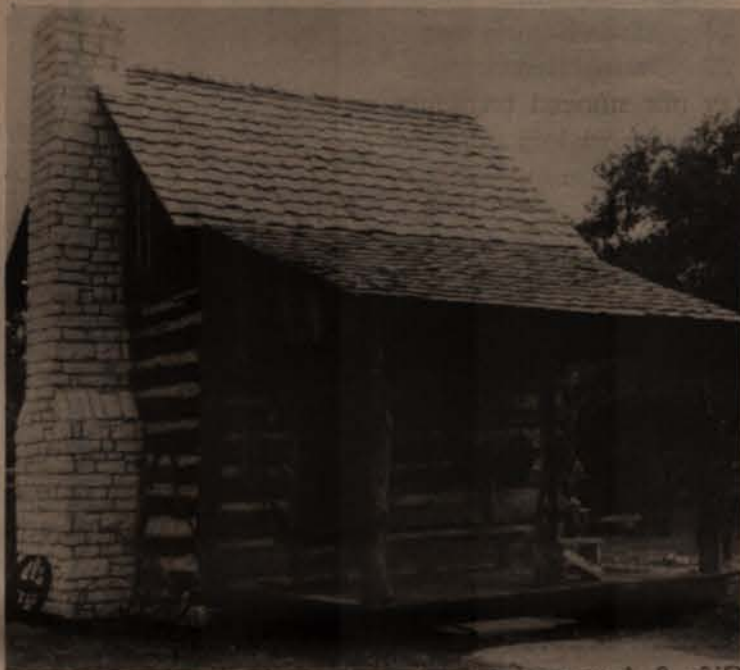
After: The restoration is complete and the old log cabin is now available for lodging at the Rose Mansion, 947-5999.
