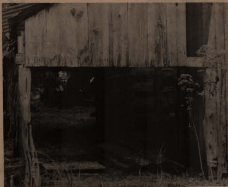
Before: This log structure was discovered under a standing wood barn. It was dismantled, moved to Salado from Little River and restored by Tommy Dean.
