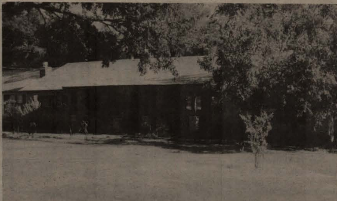
Home of Ted & Sue Edens to be featured Dec. 5-7 sits on former Indian camp ground
