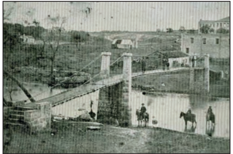
This was the first bridge across Salado Creek, built in the late 1860s.
