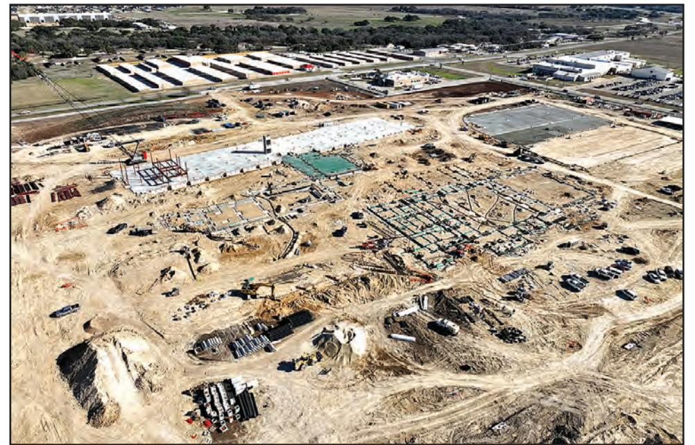
Aerial view of high school and stadium construction.
